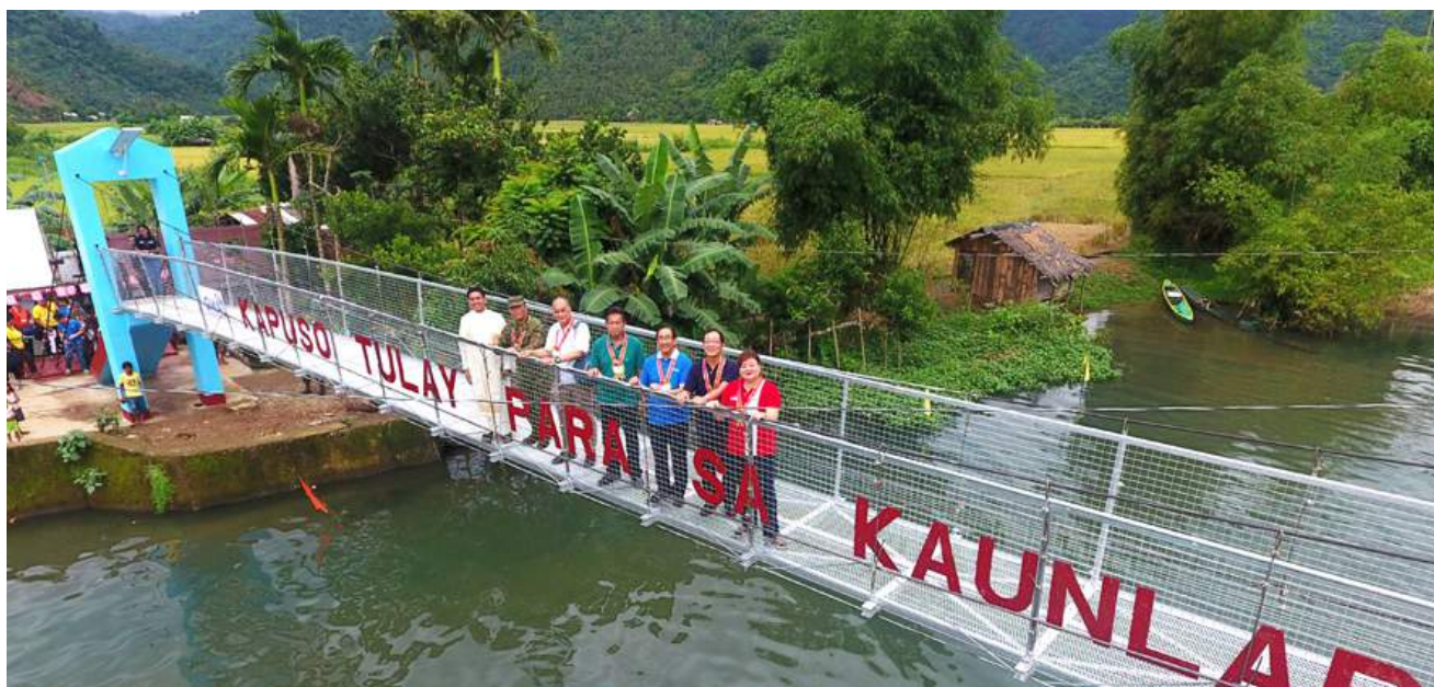
The “Kapuso” bridge was built using Republic Cement’s Rapidset cement.
